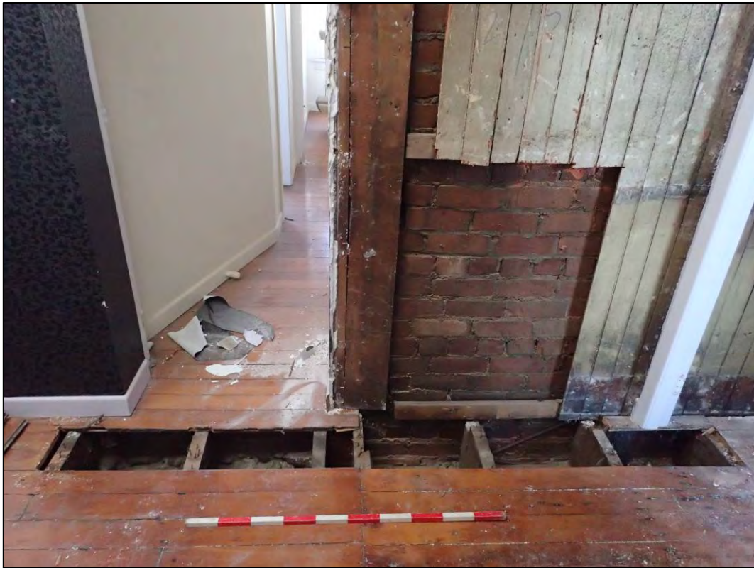
Figure 3. Sample Area showing different joists between original building extant and closed in rear stair area.
