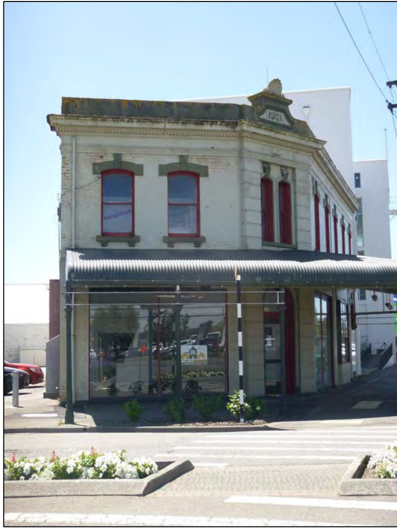
Figure 5. South elevation of 128 Main Street, Gore (Ross 22/1/2019).
