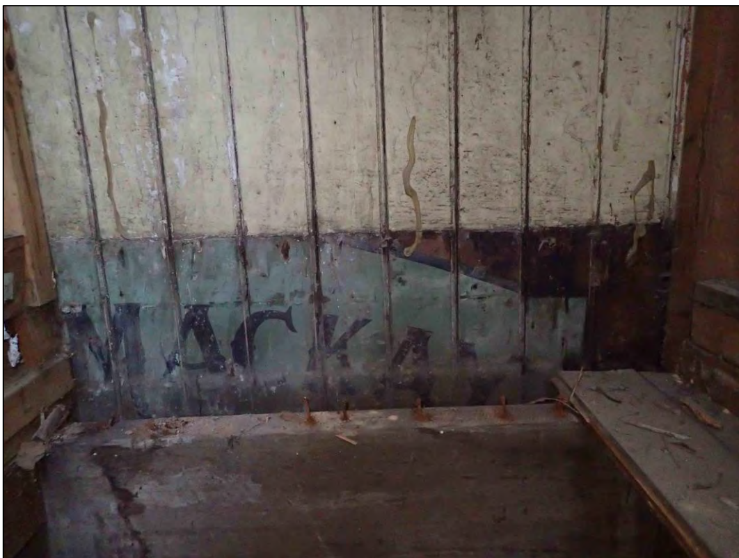
Figure 4. Mackay signage on wall, of the original building.
