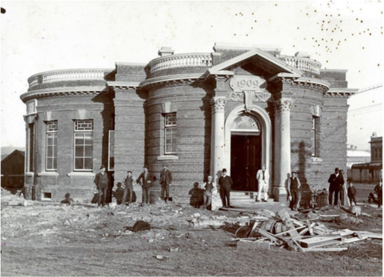
The library under construction, 1910. Gore Historical Museum.
