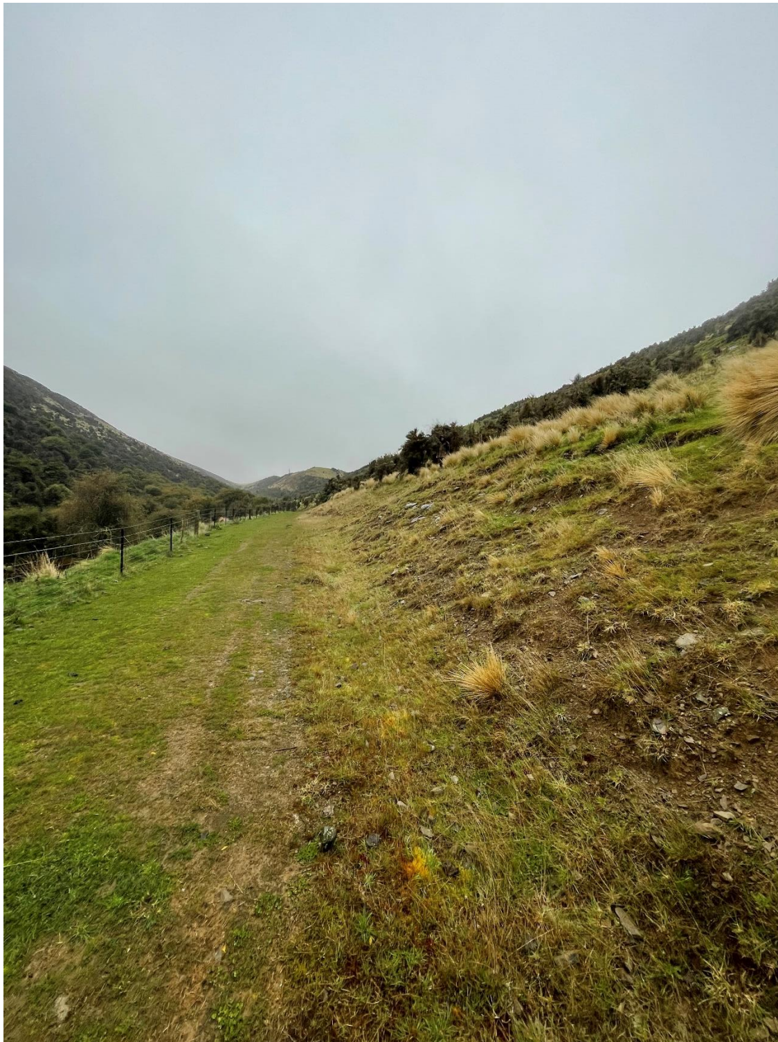
Photograph C: A 6m high cut in the internal parts of Stoney Creek Station. The batter has been laid back at 27° and has revegetated well despite minimal effort.
