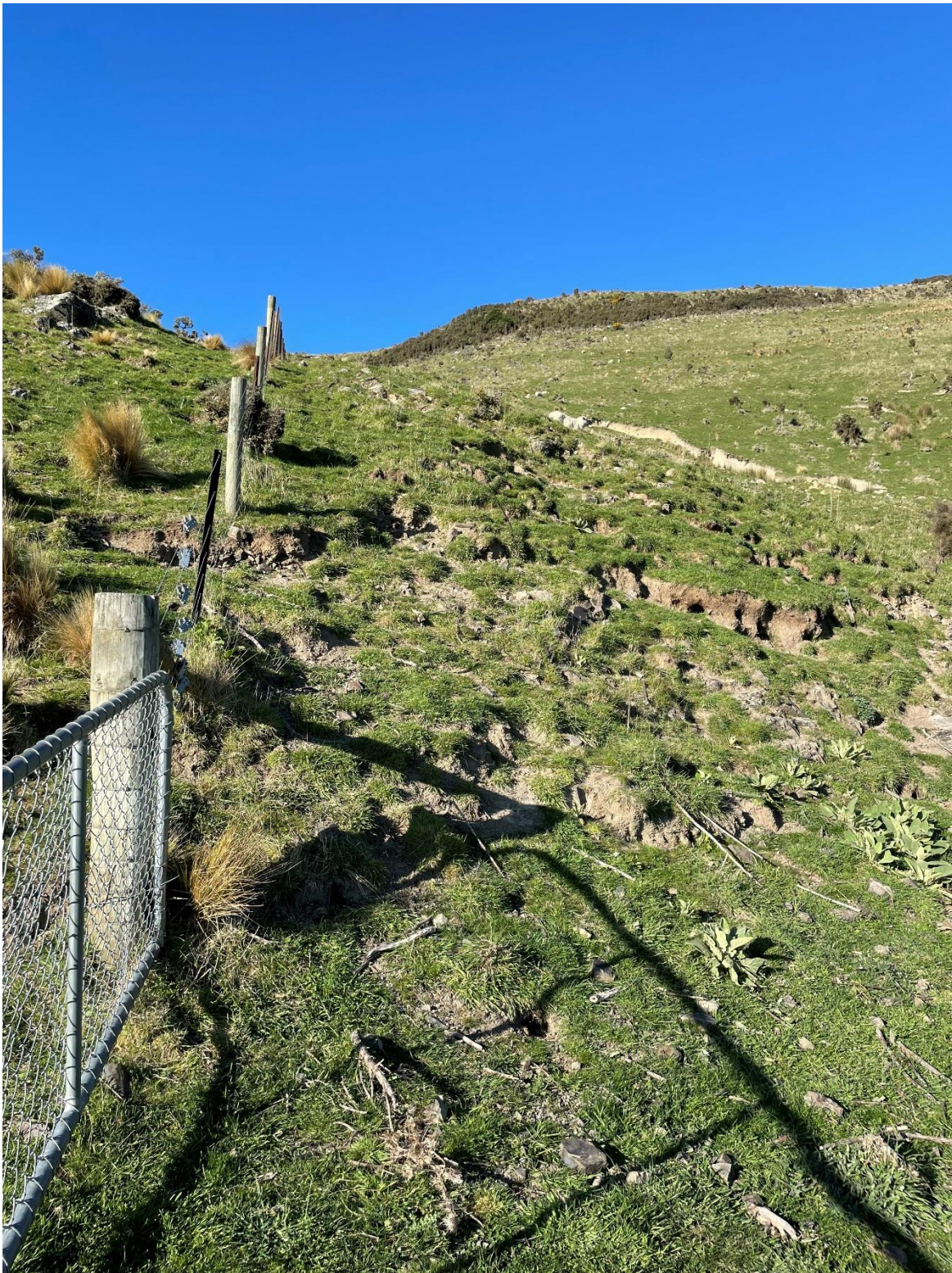
Photograph G: A 5m high cut in grazed paddock near the central northern part of Stoney Creek Station. Minimal deliberate rehabilitation has been done and batters have re-grassed naturally.
