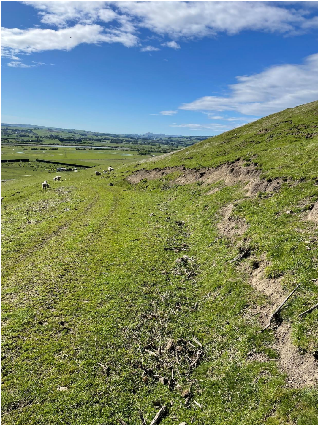
Photograph A: A 2m high cut in grazed paddock at the northeastern end of Stoney Creek Station on the front face of the hills overlooking SH94. The cut was made with minimal deliberate rehabilitation and has re-grassed naturally.
