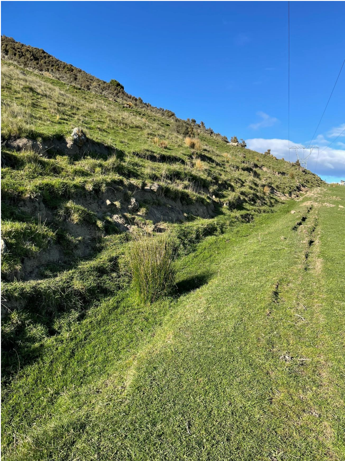
Photograph E: A 3m high cut in grazed paddock near the northwestern end of Stoney Creek Station overlooking SH94. Again, the cut was made with minimal deliberate rehabilitation and has re-grassed naturally.
