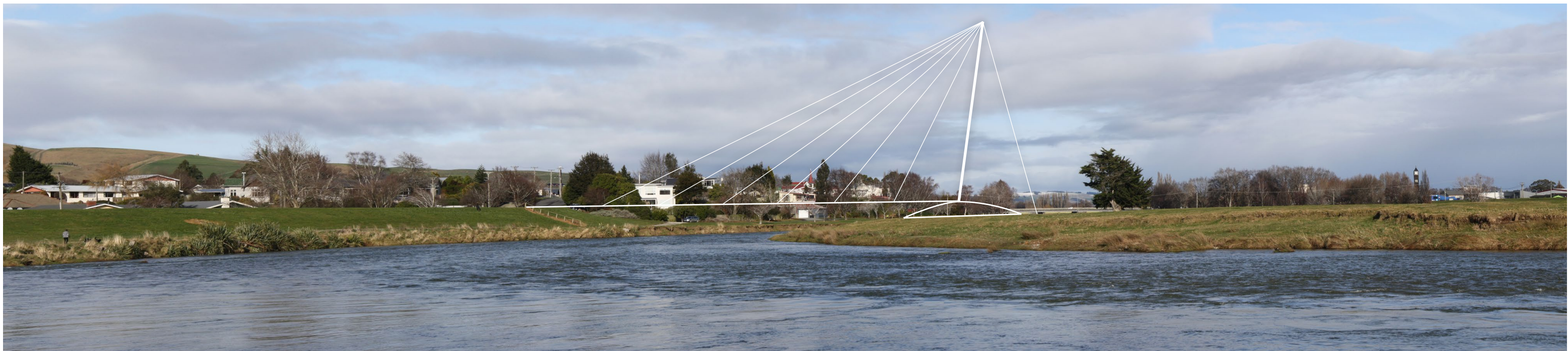
Figure 2: View toward the proposed bridge site from the picnic area adjacent to Woolwich Street, approx. 260m to the north of the bridge site.
