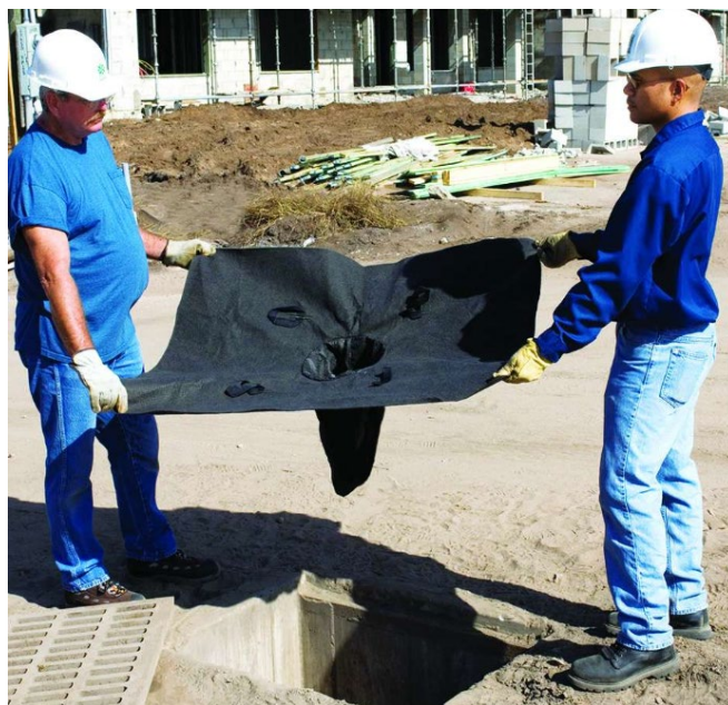
Photo 5 – Temporary drain guards that can be installed in stormwater sumps
