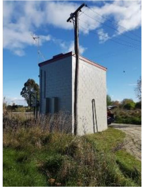
Figure 3: Otama Pump Station
