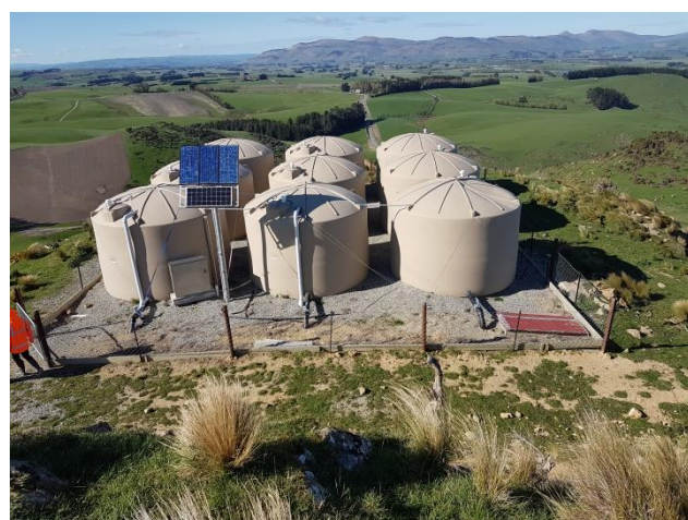
Figure 9. Pyramid Rd tank farm (9 x 25,000L)
