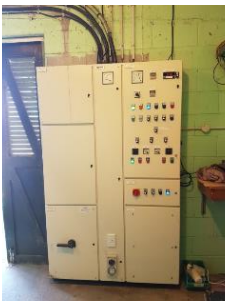
Figure 8. Pump control systems
