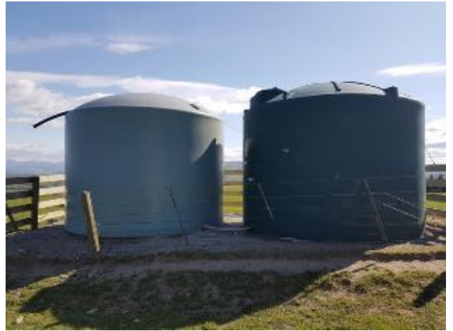
Figure 73. Barrds Break Tank
